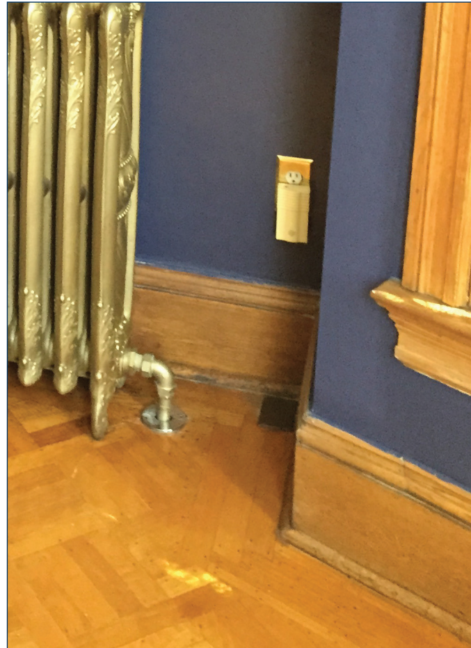
After plaster repair and painting, there is no sign that extensive piping repairs were made behind this wall.
