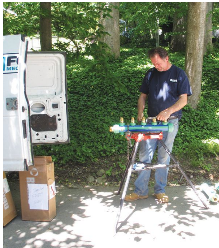
Foley Mechanical's lead technician, Dragon Vucelja, prepares a geothermal manifold for installation in a mega home.
