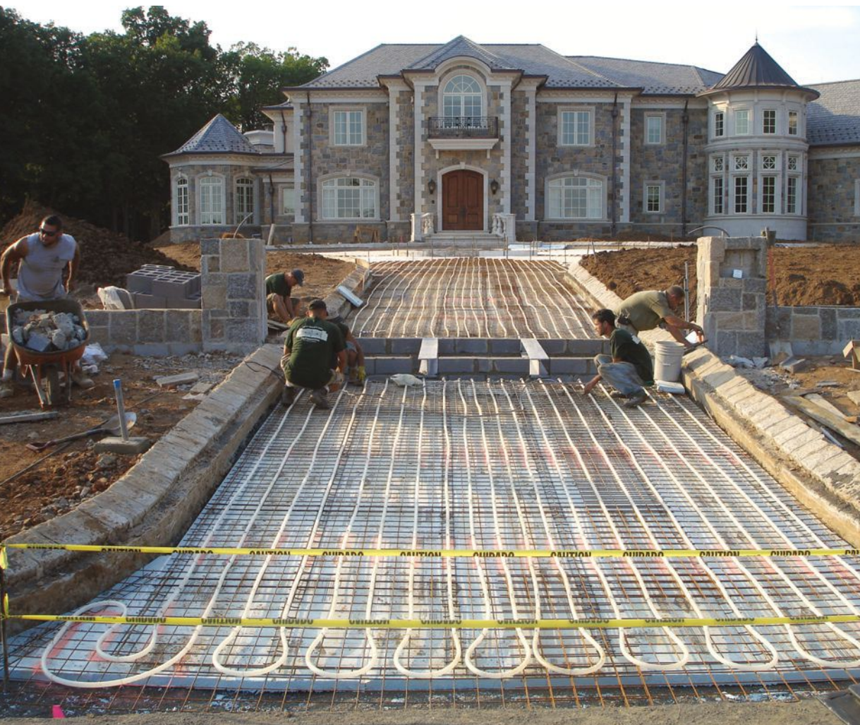
Lead technician Harvey Youker of Foley Mechanical connects ½-inch PEX tubing to a manifold on a new home in Warrenton, Virginia.
