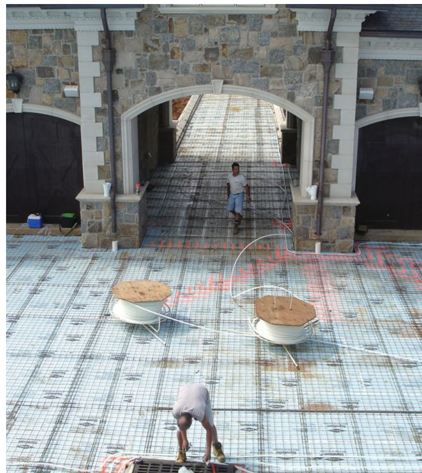
Above: Mega homes often include the installation of a snow-melting system. Left: A grand home deserves a grand snow-melting system beneath its driveway. (Photos courtesy of William Jannone & Sons Inc.)
